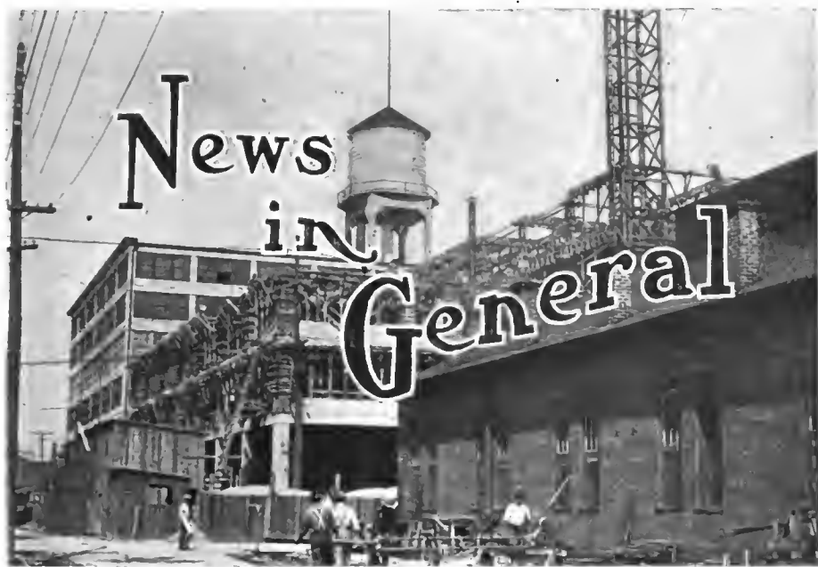
Six-Story Addition to Stoddard-Dayton Plant, Now Building
